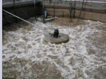
Fig. 4. FOG and foam reduction using BioFOG 3205.
