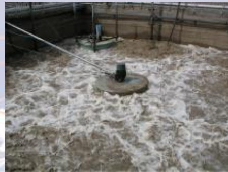
Fig. 4. FOG and foam reduction using BioFOG 3200.
